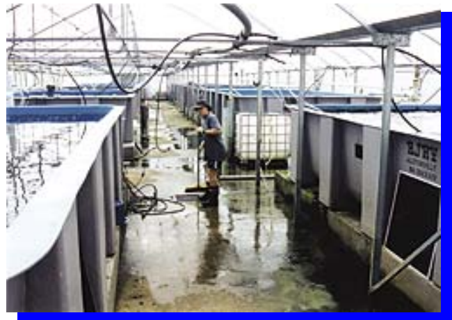
The 10 x 30,000-liter barramundi tanks in the twin-span polyhouse at Tailor Made Fish Farms Pty Ltd., Port Stephens, near Newcastle, New South Wales. The 10 tanks have the capacity to produce at least one ton/week. Current harvest is 600 kg/week.
